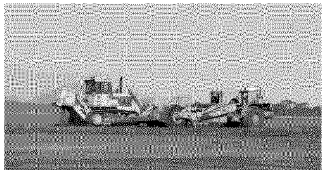
Dozer and Scraper
