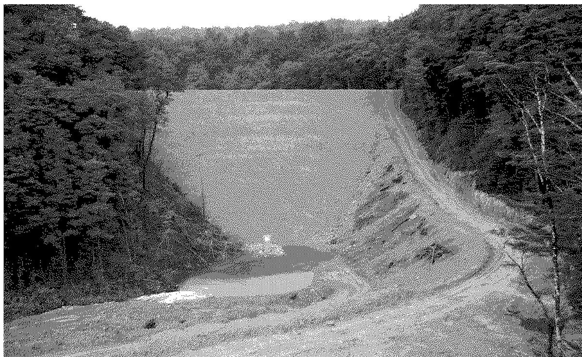
- Figure 1 - Fossicker's Creek Tailings Dam Globe Progress Project
