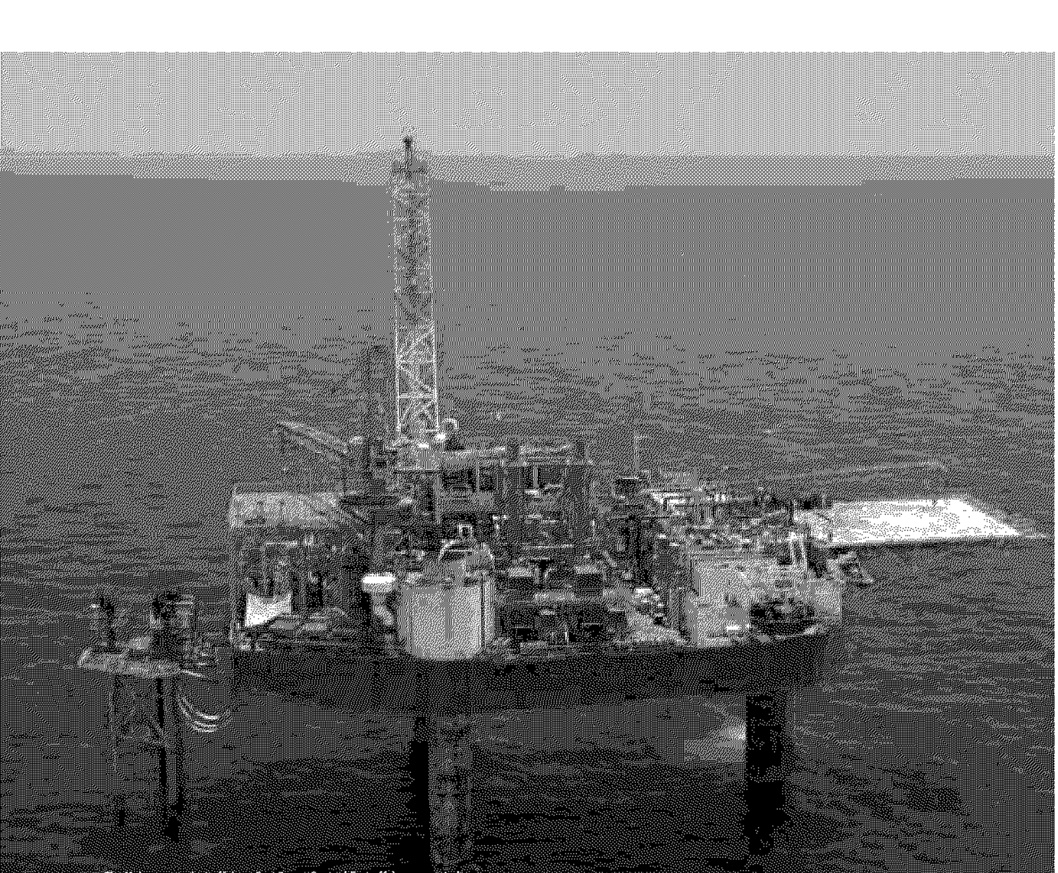
The Maleo gas project offshore East Java – Santos' first offshore operated gas field outside Australia – started production in September 2006.
