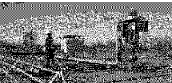
Sustainable practices at the Cooper Basin Oil Project, south-west Queensland. Top: Tarbat camp housed under a large verandah which reduces energy use and creates more comfortable conditions for employees. Centre: Installation of environmentally-friendly glass-reinforced epoxy flowlines. Bottom: Completed oil wellhead, including energy-efficient progressive cavity pumps, solar-powered telemetry and guards to protect local livestock.
