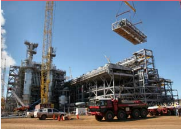
Train 5 modules being assembled
