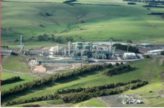
The Otway gas plant near Port Campbell, Victoria.
