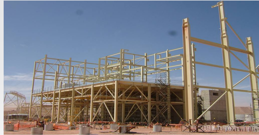
Grinding area structure
