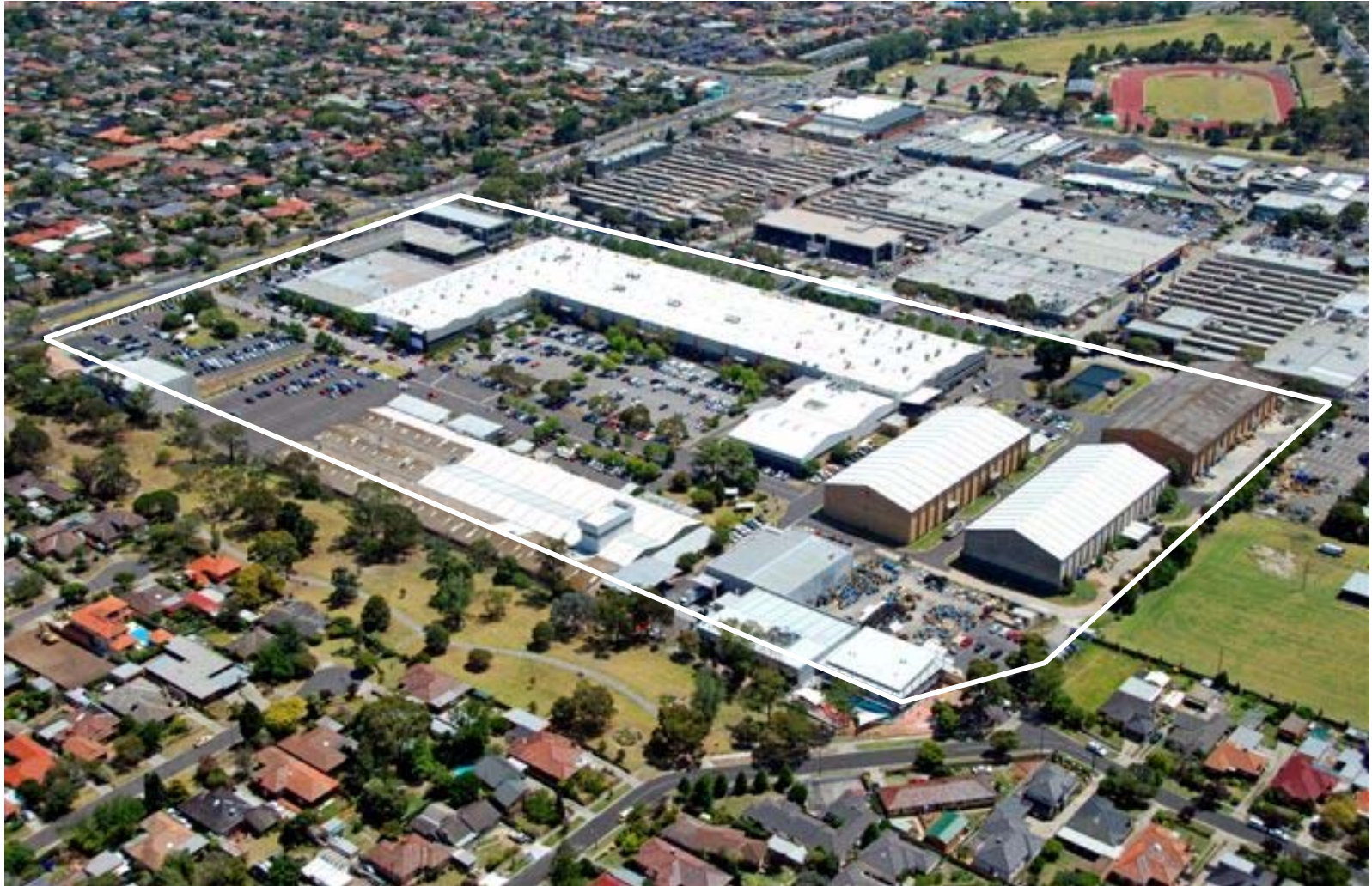
Virginia Park, 232-262 East Boundary Road, Bentleigh East, Victoria
