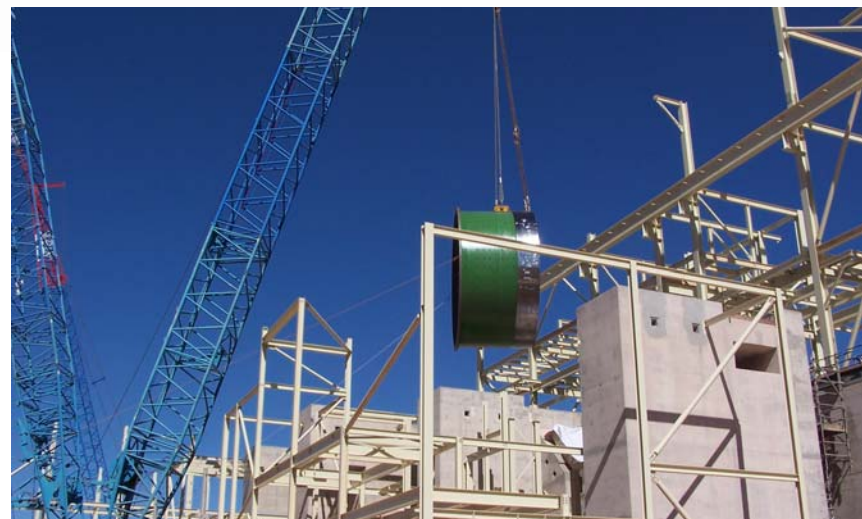
Ball Mill installation
