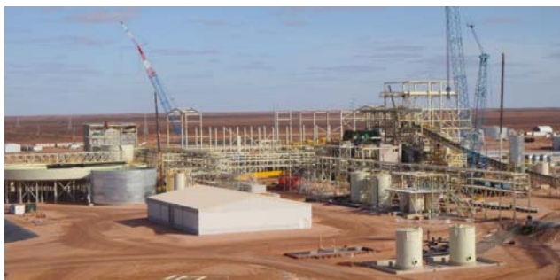
Overall construction at Prominent Hill is 72% complete.
