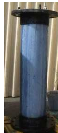
Liner being pressure tested
