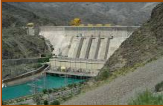
Hydro power station
