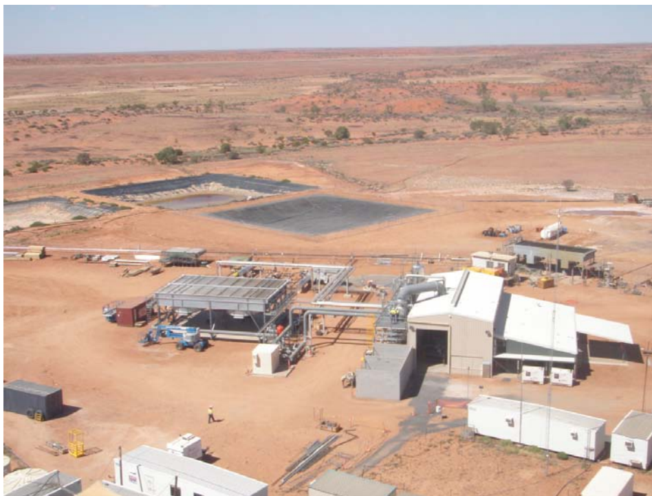
Aerial view of the 1 MW Pilot Plant and Visitor Centre
