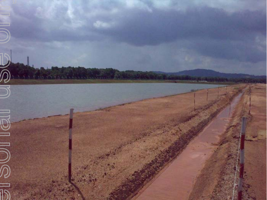
Lynas-constructed stormwater detention pond
