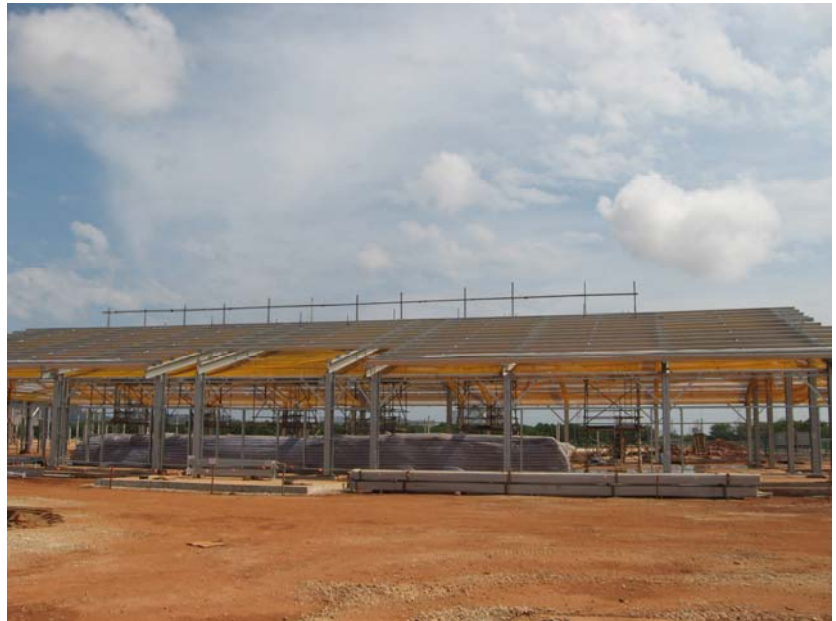
Building construction has commenced
