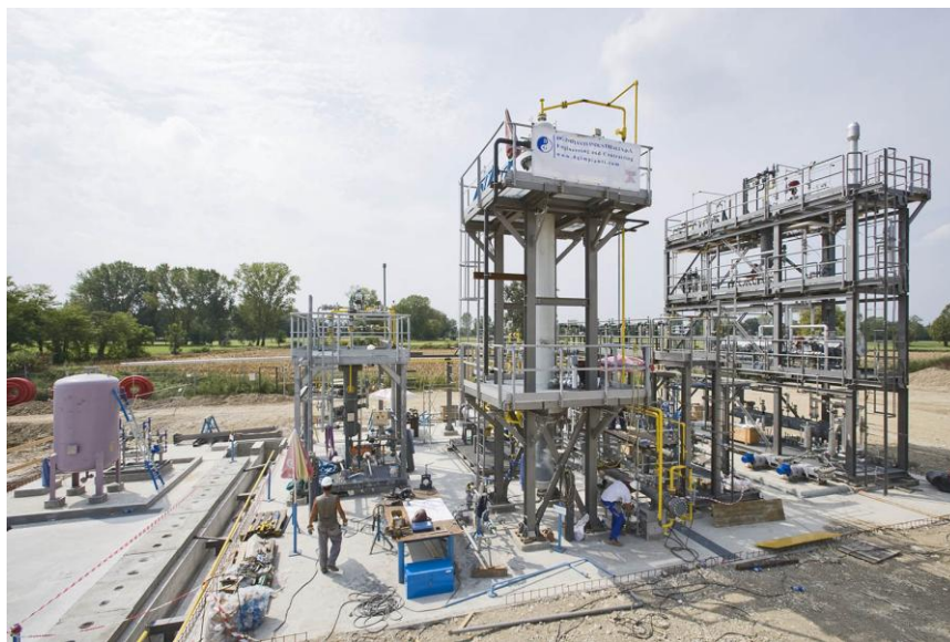
Installation works at the Castello gas field
