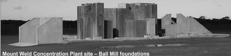
Mount Weld Concentration Plant site – Ball Mill foundations
