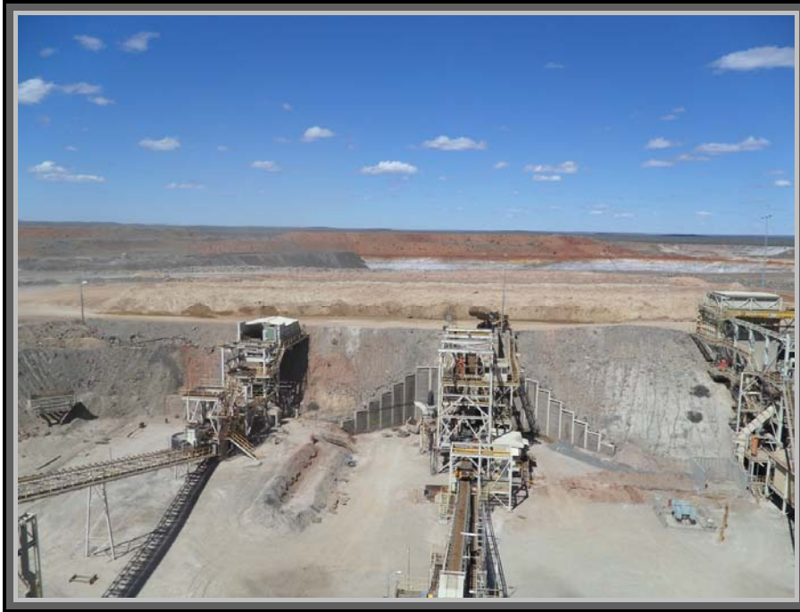
View of BGSM RoM pad and primary crushing facilities
