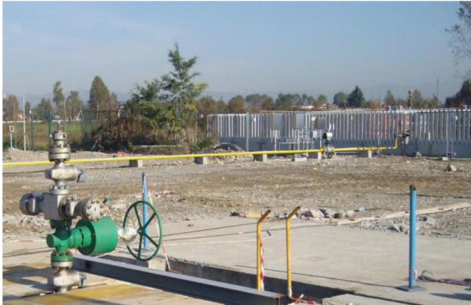
Pipeline ready at Castello gas field
