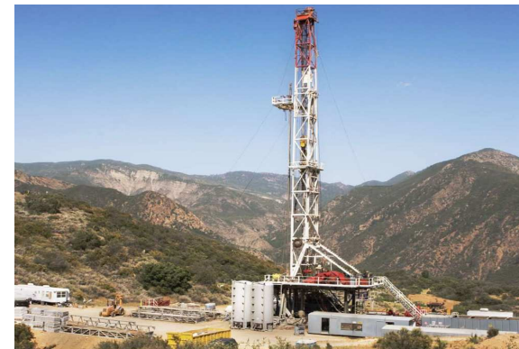
Drilling the Nesbitt -5 well at the Silverthread project
