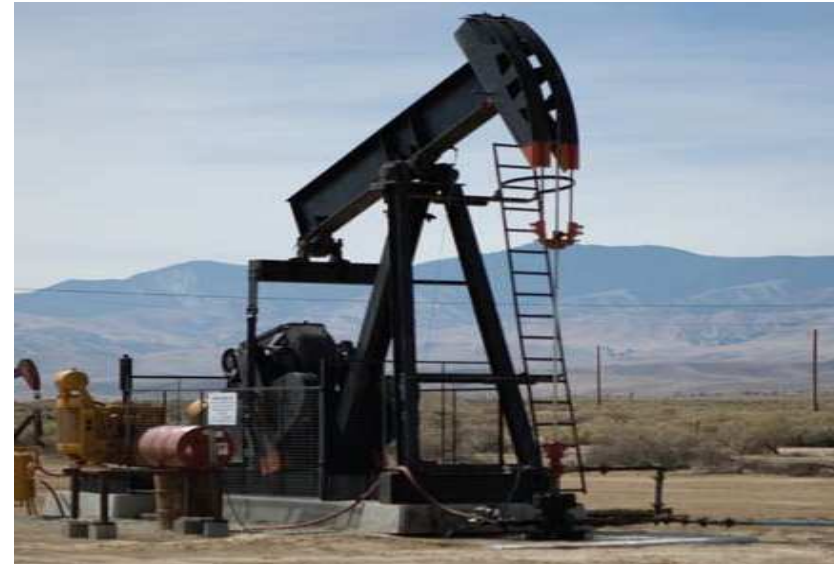
Beam pump on oil producer Maricopa - 6
