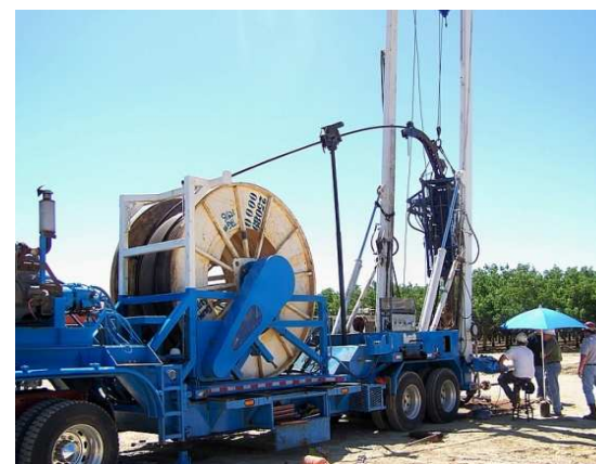
Coiled tubing unit in operation at SELH during well workover
