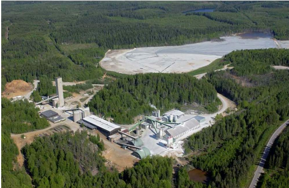
Luikonlahti Processing Plant and Tailings Dam
