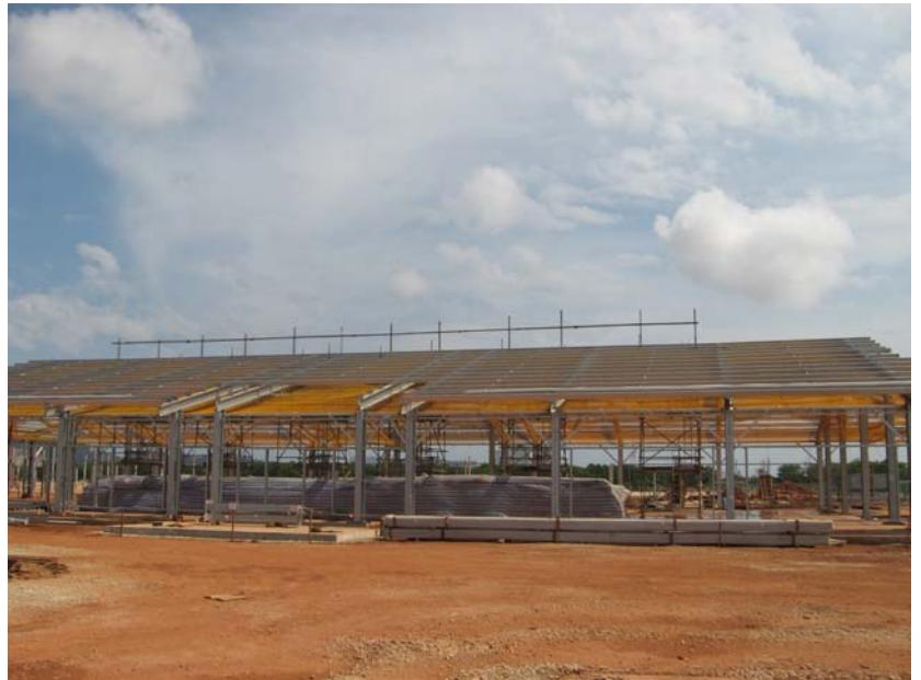
Building construction has commenced
