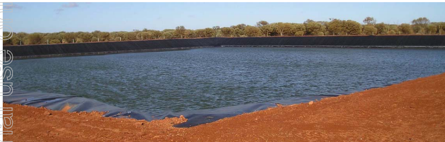
Process water treatment pond complete
