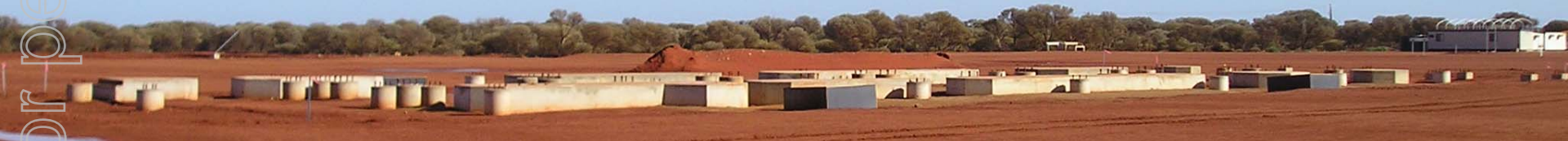
Mount Weld Concentration Plant site – Flotation Plant foundations
