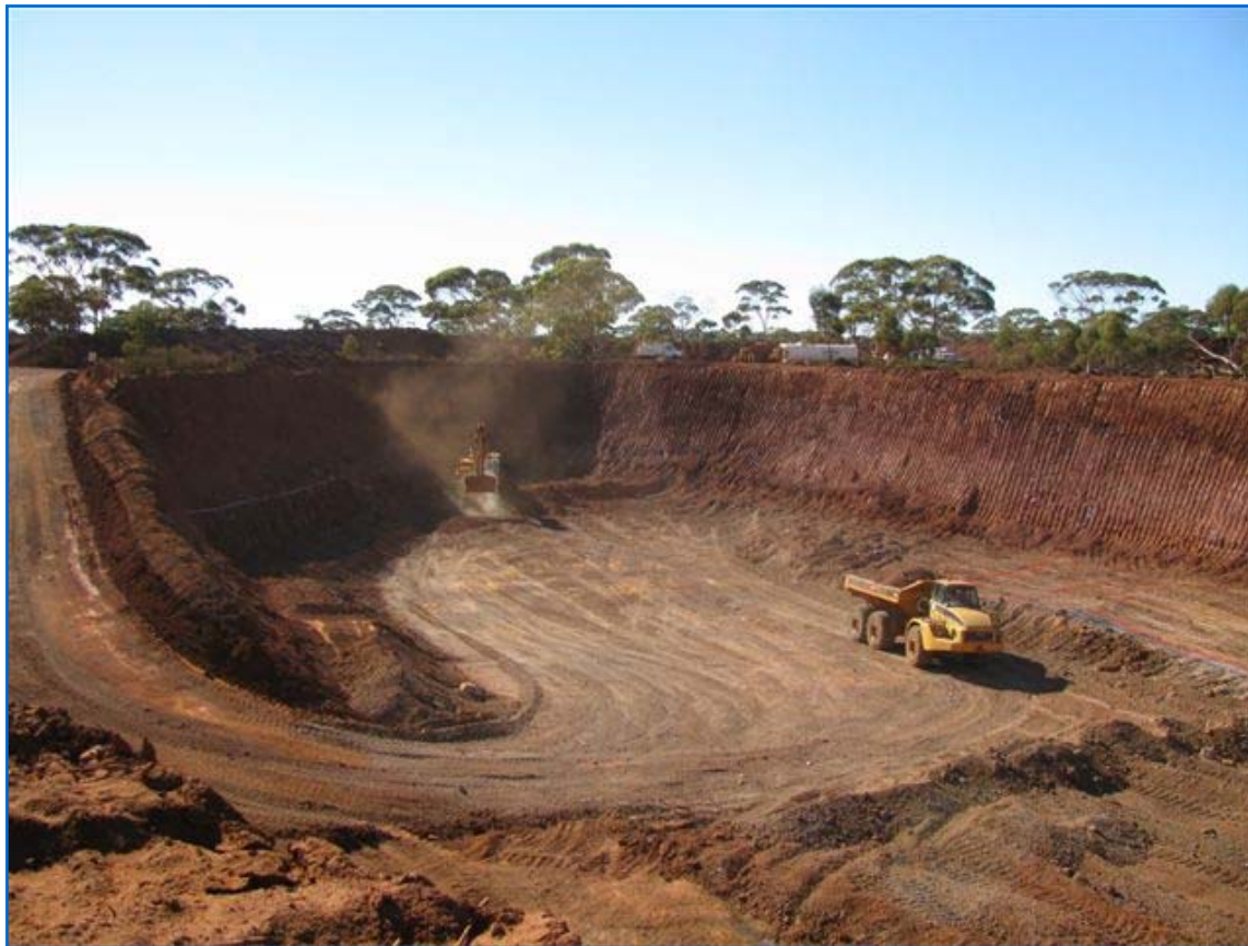
Typical oxide open pit as will be mined at Cardinia
