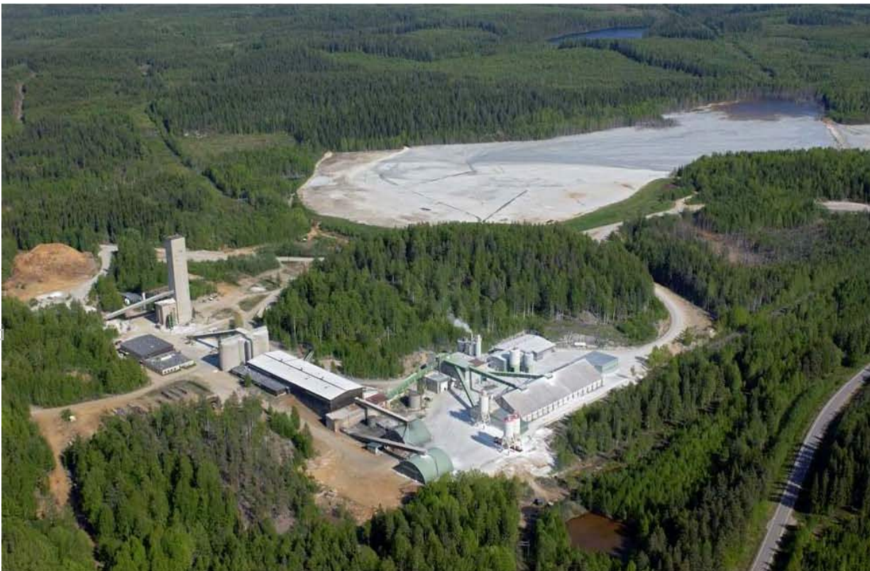
Luikonlahti Processing Plant and Tailings Dam
