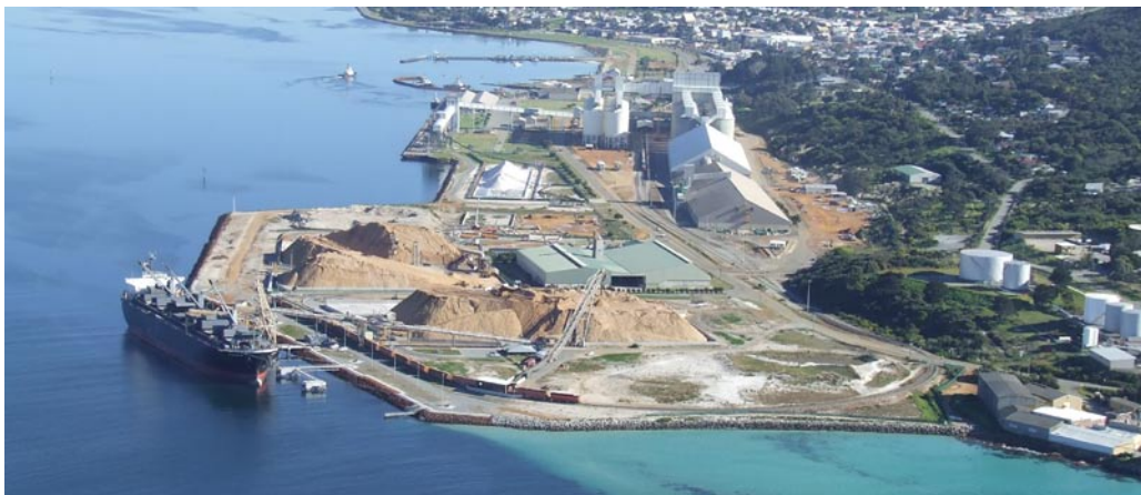
Figure 1 - Albany Port showing proposed location of new Berth in foreground.
