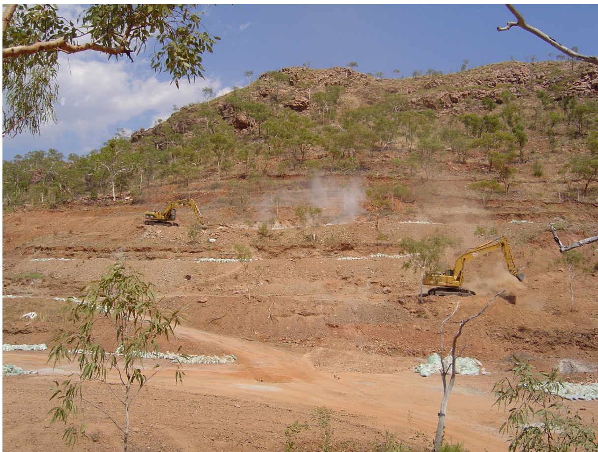
Figure 1: Rehabilitation work concluding the resource drilling at Eva
