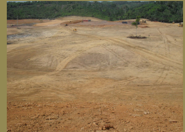
Plant site access road
