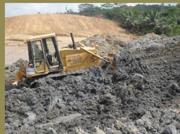
Mining Office setout
