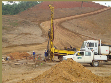
Geotech Drilling – Thickener Area
