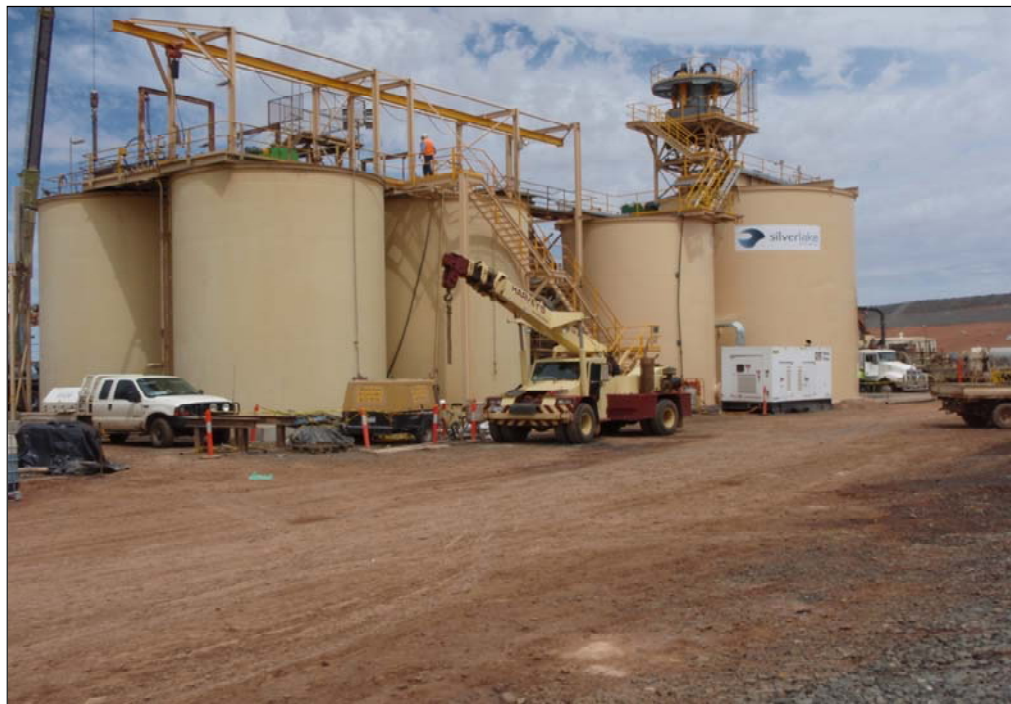
600,000 tpa Lakewood Gold Processing Facility
