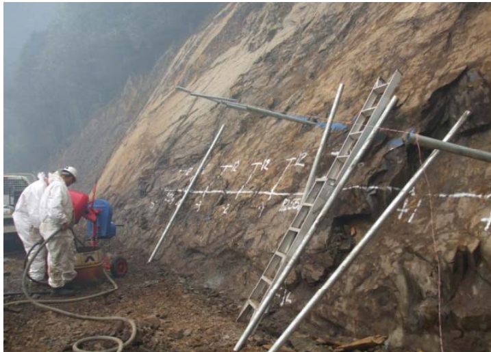
Installing ground support for Decline portal
