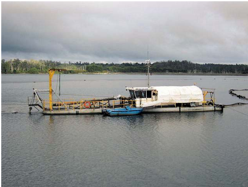
Bass' dredge on Hellyer Tails Dam doing rehab. In Jan 2010
