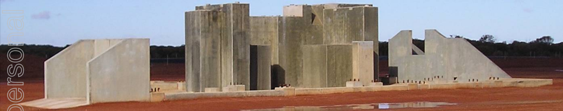
Mount Weld Concentration Plant site – Ball Mill foundations
