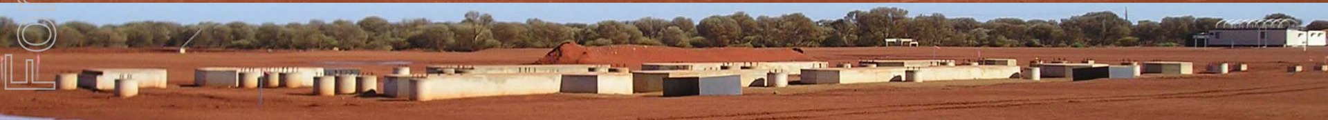
Mount Weld Concentration Plant site – Floatation Plant foundations
