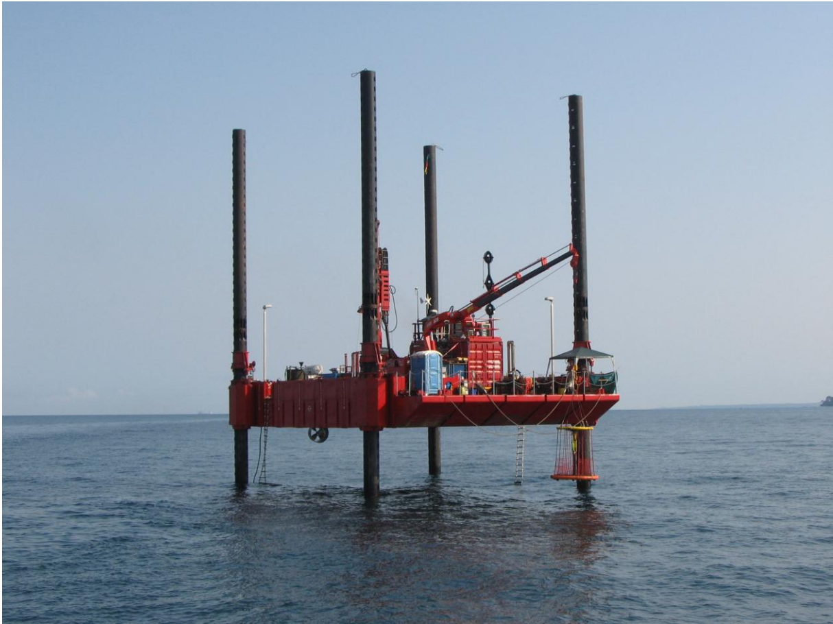
Figure 3: Offshore Drill Rig operating at Lolabe Port
