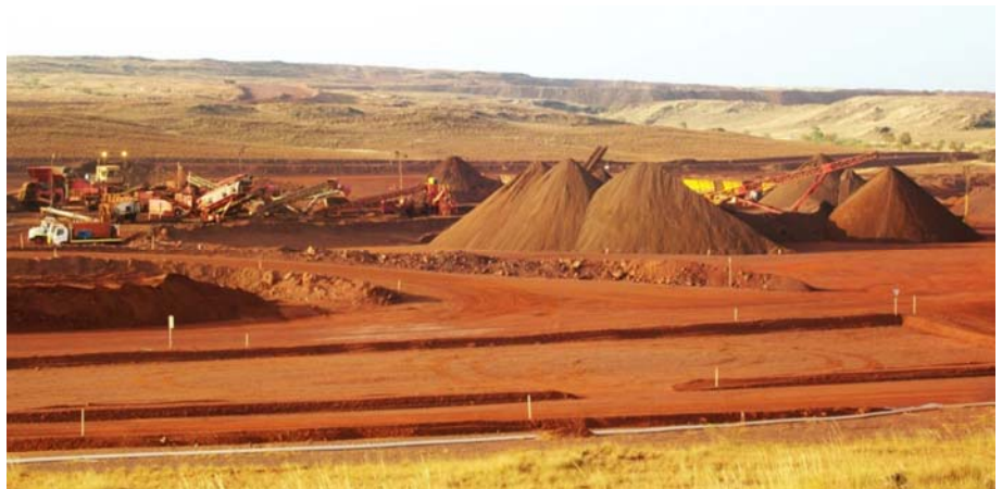
Figure 1: Upgraded DSO crush and screen plant at Pardoo capable of 2.4Mtpa
