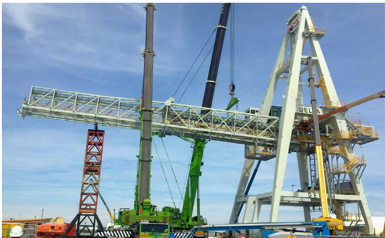
Figure 6: Utah Point Shiploader being assembled
