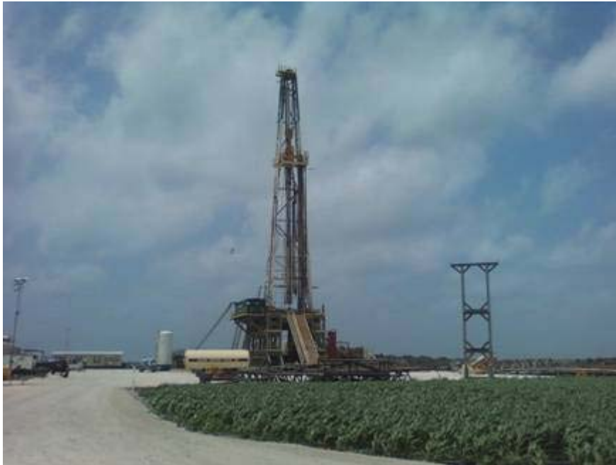
Figure 2: Precision #37 rig drilling ahead on Russell Bevly #1 Well
