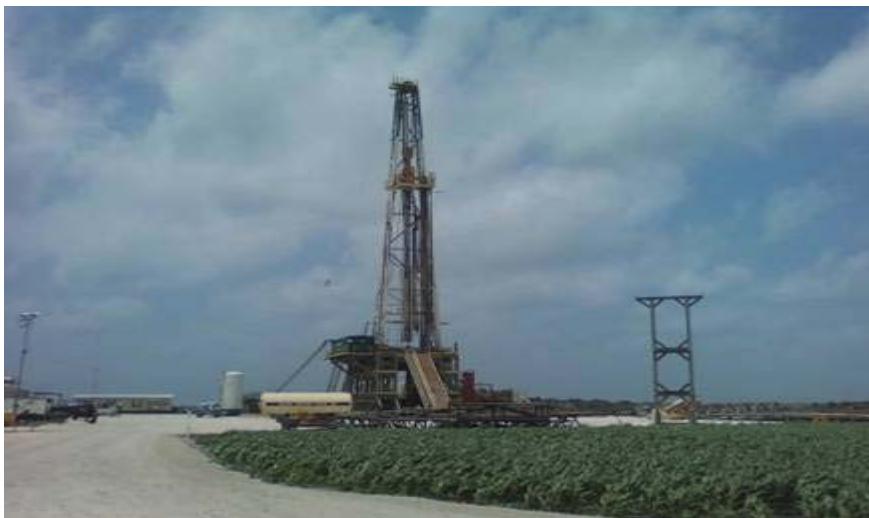
Figure 1: Precision #37 rig drilling ahead on Russell Bevly #1 Well
