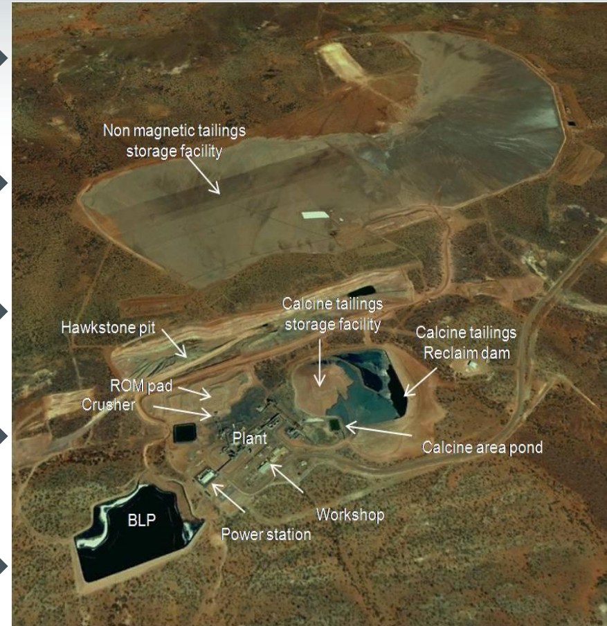
Aerial view of Windimurra mine and plant
