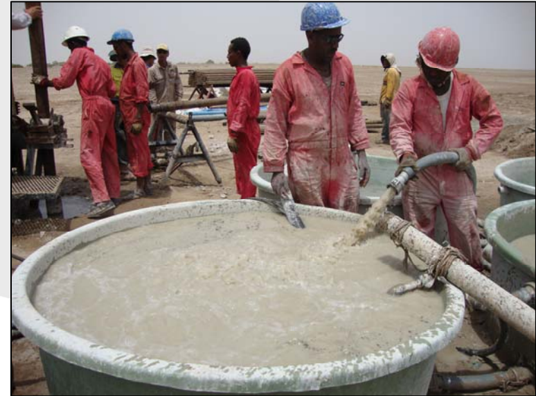
Above; South Boulder crew checking the important drilling mud. Below; South Boulder Geologist examining some of the first the potash core.
