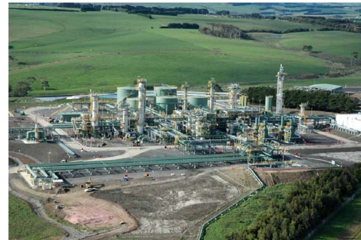
Otway onshore production facilities
