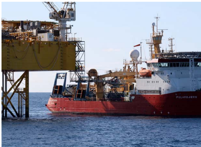
Maintenance activities being undertaken at BassGas
