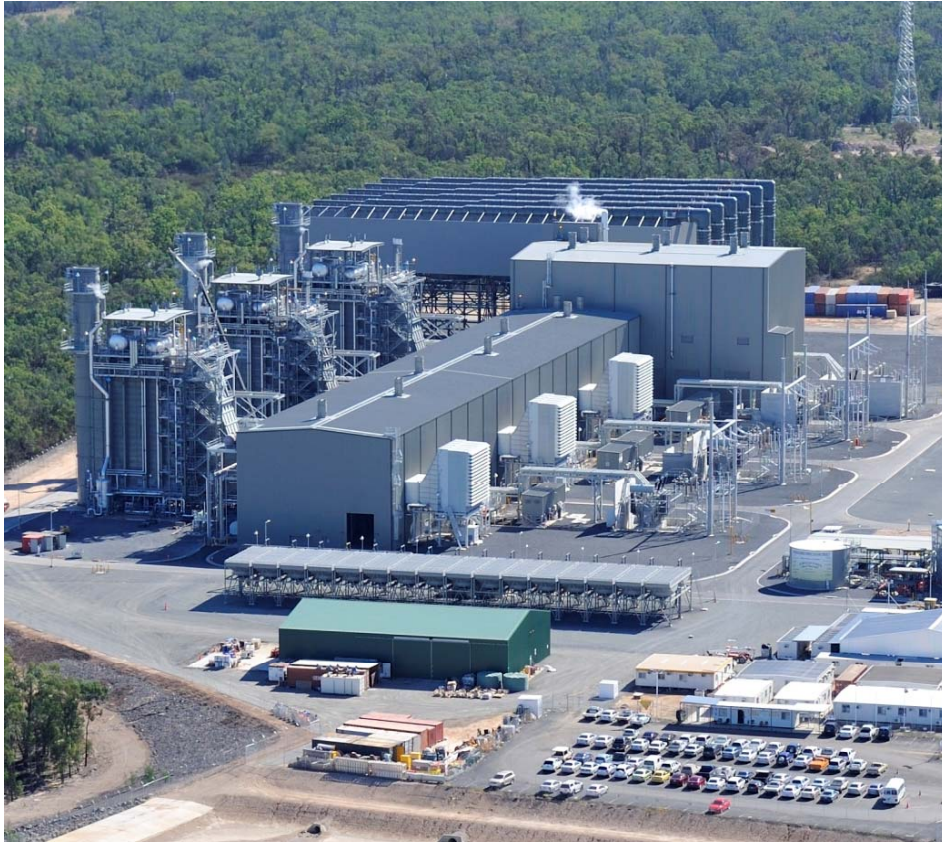
Darling Downs Power Station
