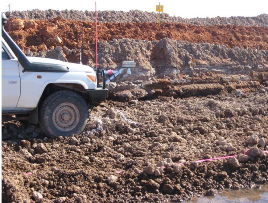
Figure 3: Vehicle mounted Gamma logger for pit floor grade mapping
