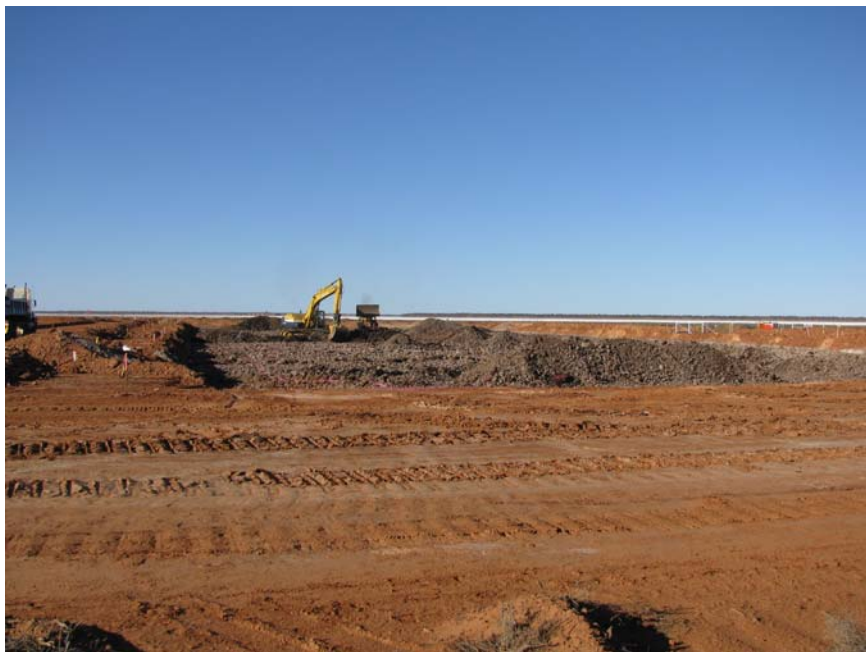
Figure 2: Excavator and loader selectively removing waste and mineralised material for stockpiling
