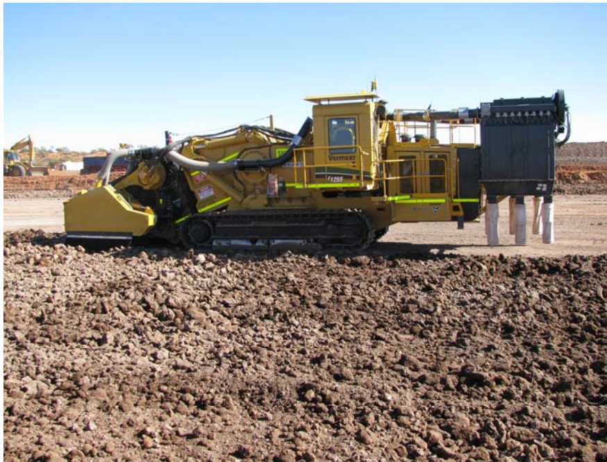
Figure 1: Vermeer machine cutting pit floor
