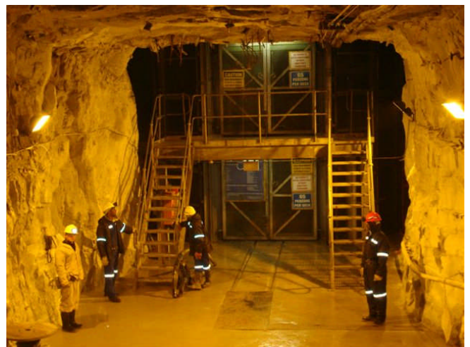
BPLZ Level Station
