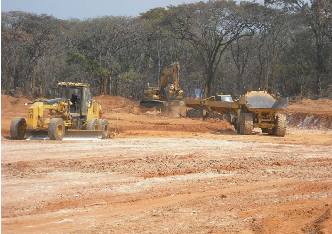
Plant site earthworks – Kipoi Stage 1
