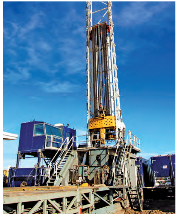
Boomerang Well drilling
