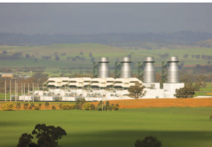
Uranquinty Power Station near Wagga Wagga, New South Wales
