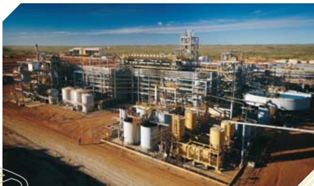
Telfer Processing Plant
