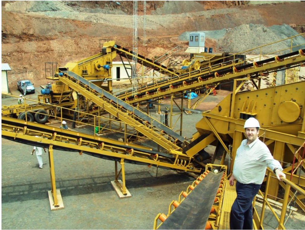
Figure 1: Crusader Company Secretary, Andrew Beigel, inspects the Posse beneficiation plant.
