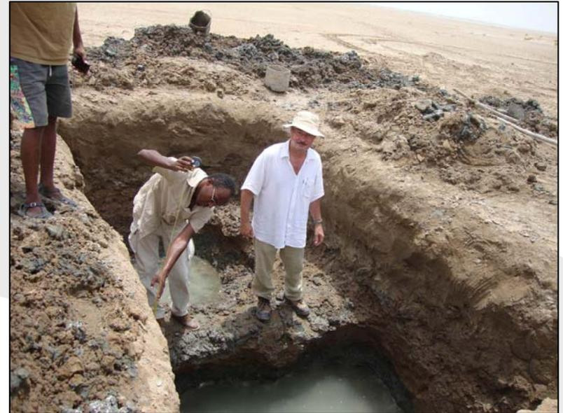
Above; Drill sumps in the salt flat provide a source of drilling water.
