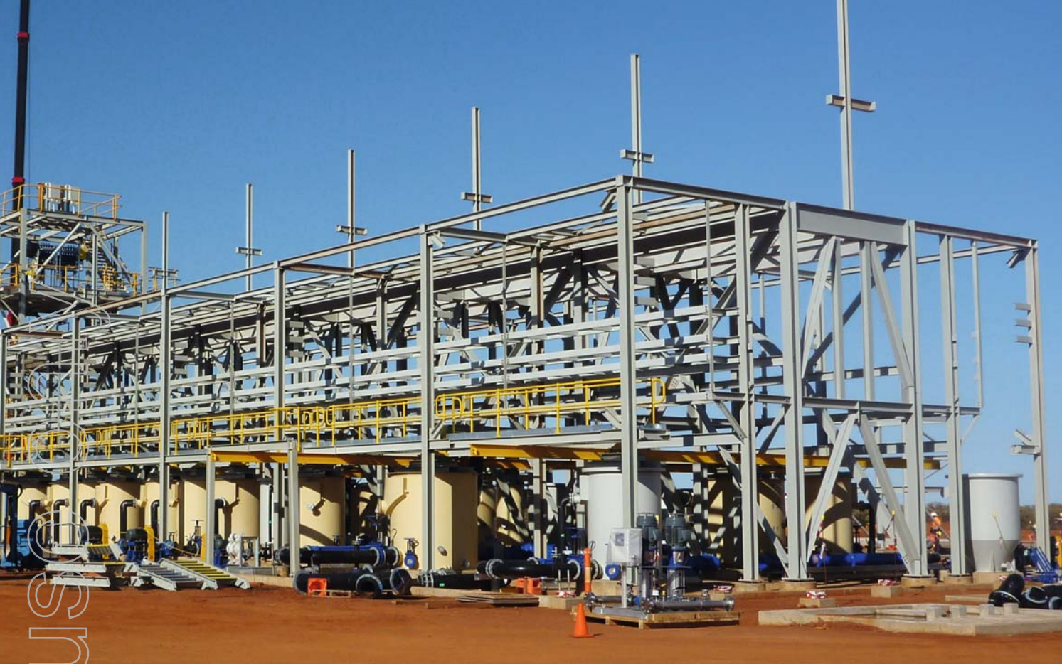
Flotation building under construction at the Concentration Plant, Western Australia.
