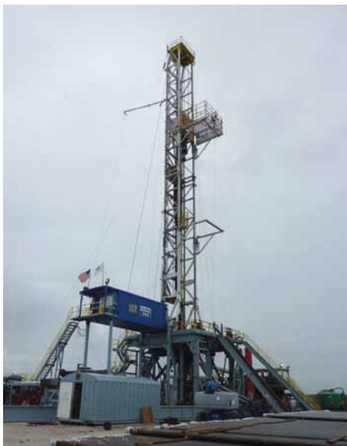
Drilling at Sugarkane
