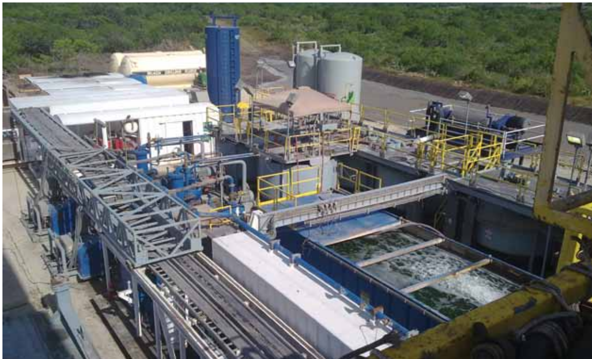
Surface operations at Rancho Grande #1
