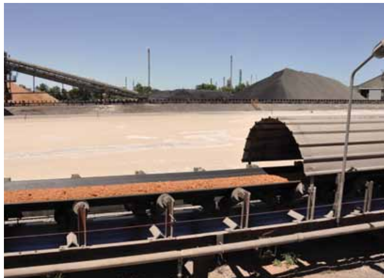
4. Bauxite ore on conveyer system for ship loading at Kwinana
