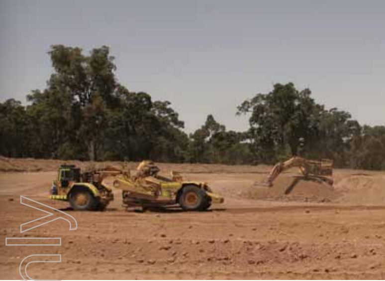
1. Bauxite extraction at north Bindoon trial operations
