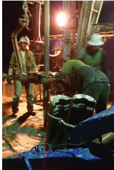
Below: Various operations in the Otway Petroleum Project during 2010
