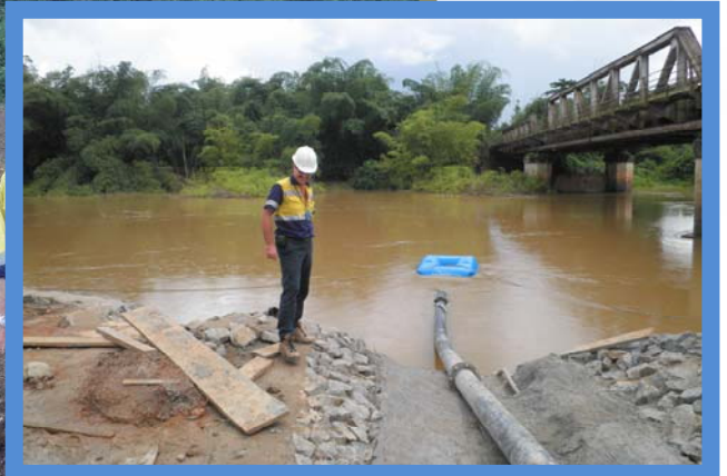
Ankobra River pump and pipeline commissioned
