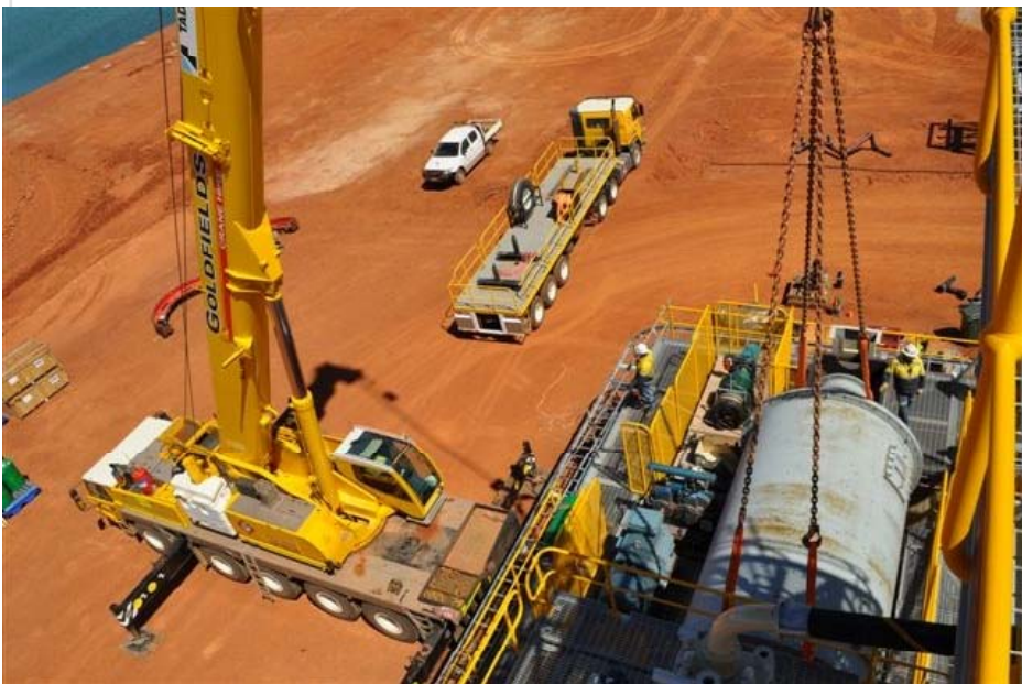
Ball mill being installed
