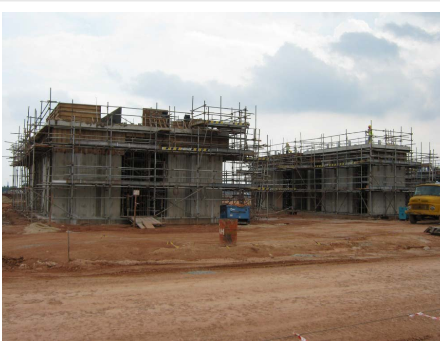
Rotary kilns foundations
