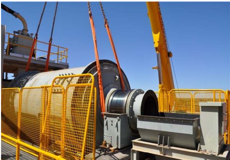
Ball mill being installed
