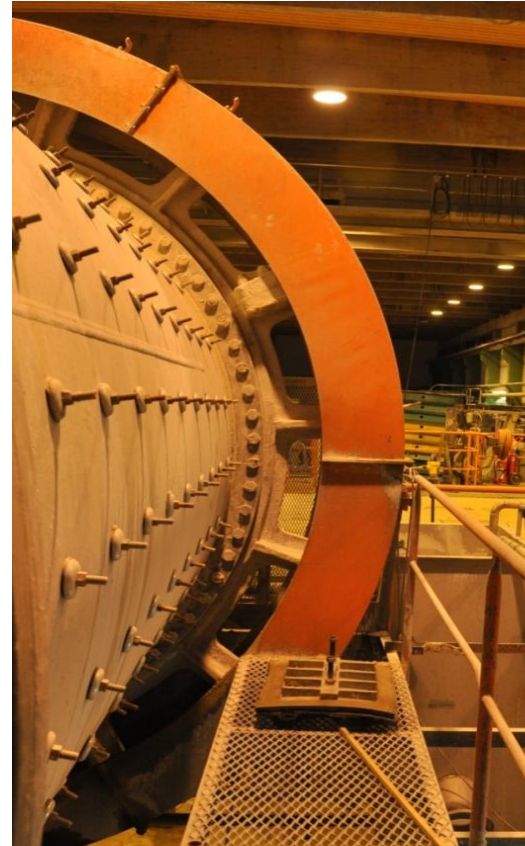
Luikonlahti Mill: Interior of flotation and grinding hall
