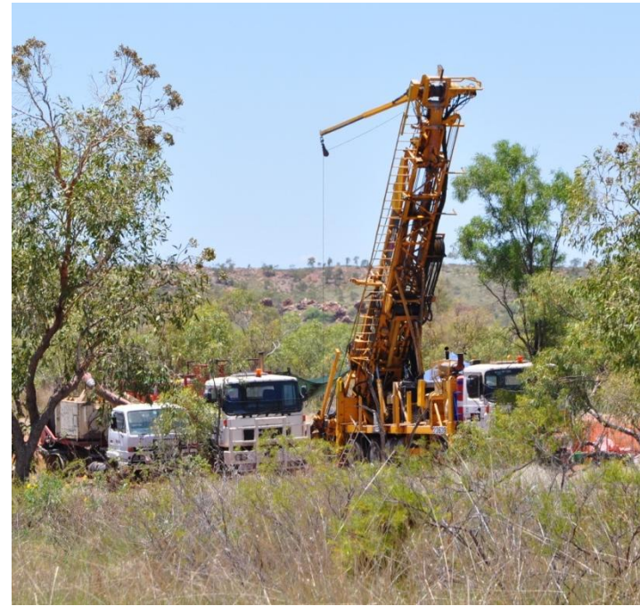
Xstrata drill rig at the Blackard deposit
